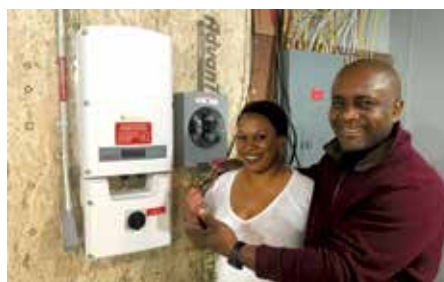
Stephen and Arlene England, Habitat homeowners in Roslindale, show off the inverter that turns solar power into electricity for their home. The Englands had an electric bill of only $10 this September.
